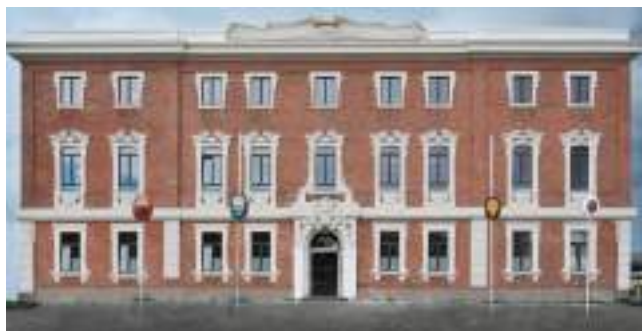
Figure 12: Magazzini Generali building
